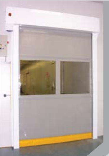
Profile rapid door in a pharmaceutical facility
